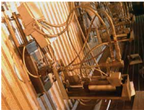
CCA SNCR Tilting Injector
