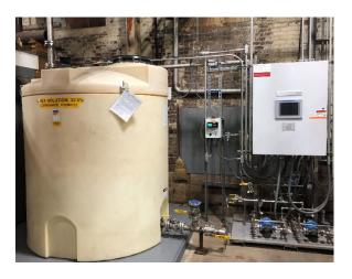
Rather than the typical multi-element ammonia injection grid, the system operates efficiently with two urea injectors through each side of the breeching.
