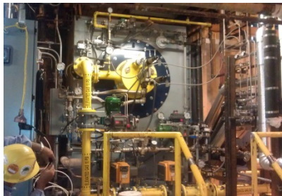
Boiler #1 with new burner installed
